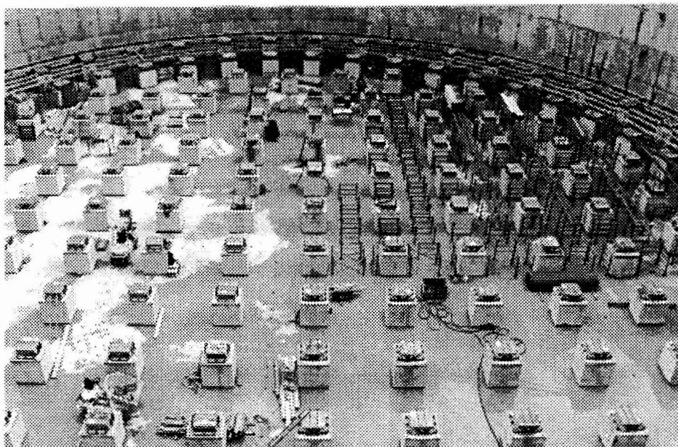
Fig. 9 Installation of Friction Pendulum Bearings
